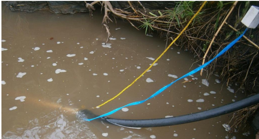
Figure 16: The submersible pump lying in the river is only fixed with the yellow rope in Morogoro region, Tanzania. April 2019.
